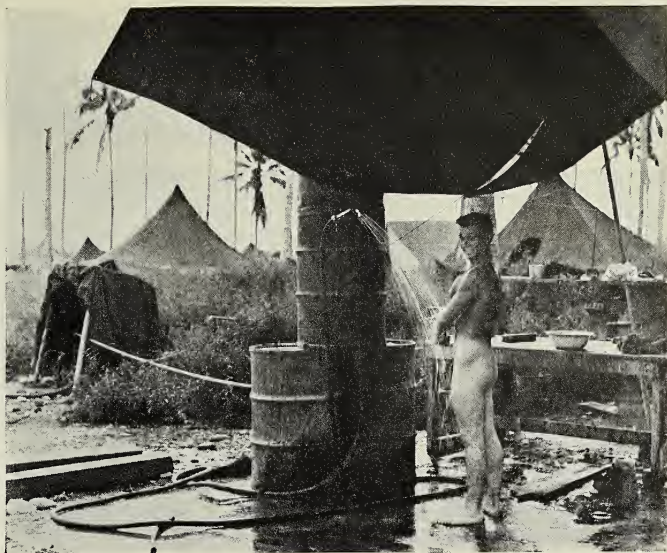
AACS shower at Henderson. Re-fueling pump produces 30 lbs. water pressure in the airtight drums.
